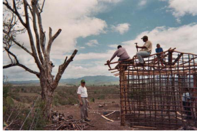
Greg Helps the Villagers With the Roof
