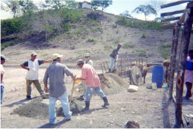
Villagers Mixing Concrete With Beth Ann
