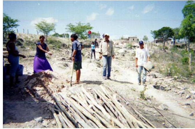
Villagers Getting Ready to Mud Some Walls
